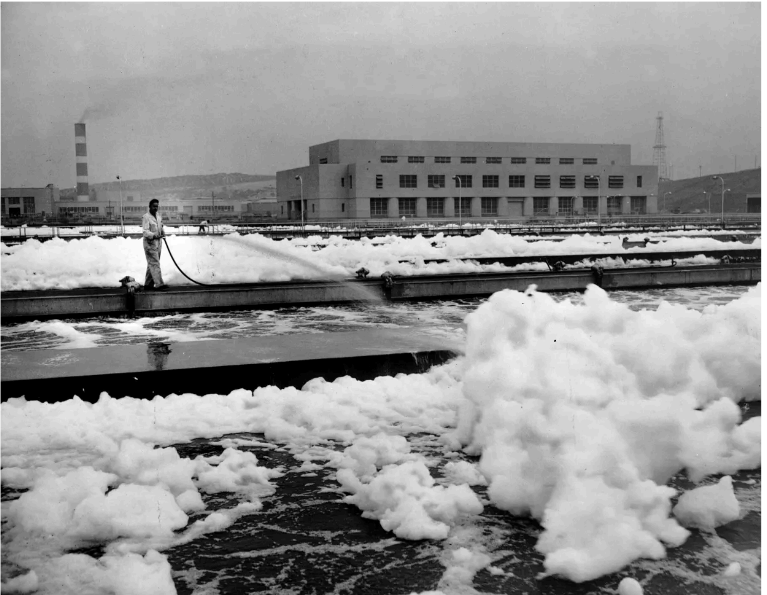
Foam forms in billowy masses and even blows over the hill to El Segundo from washing machine and dishpan suds effluent at the Hyperion Water Reclamation Plant in 1951. (Los Angeles Examiner / USC Libraries / Corbis via Getty Images)
